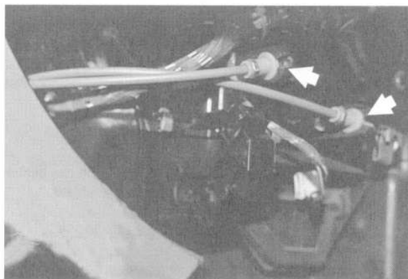
Fig. 15. Control cables for air distribution levers (arrows).
