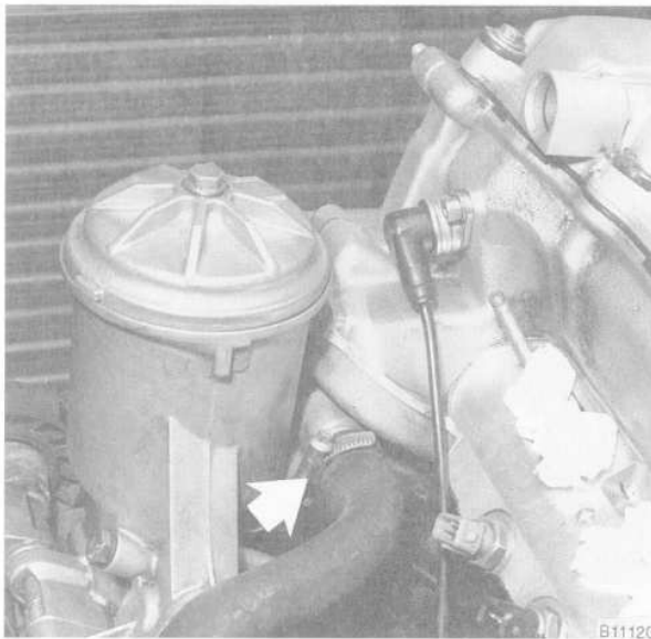
Fig. 6. Coolant hose at oil filter housing (arrow).
